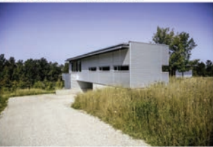
House in Mulmur Hills 3 is a composition of heavy steel, concrete, big timber beams and glass.
